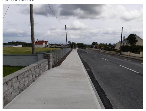
570m of footpath installation completed on the R364 at Kilkerrin along with drainage works and public lighting.
