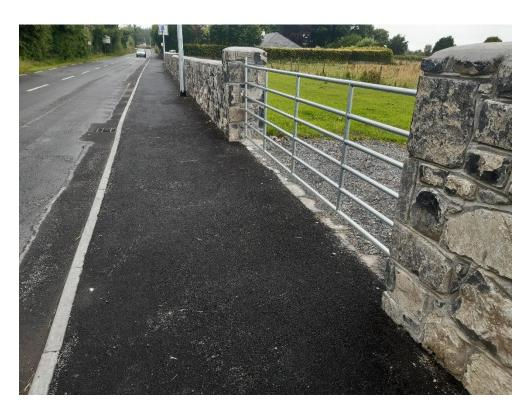
590m of footpath installation completed on the R360 at Williamstown along with wall building, drainage works and public lighting.
